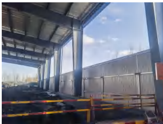
污泥堆放场围挡+罩棚
